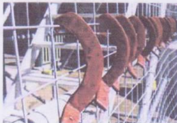
Original brackets were reinstated during works on the roof.
